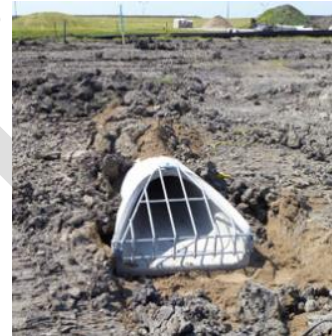
Figure 3-2 Flared End Section, ARC, Fargo, North Dakota
