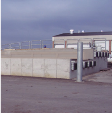
Figure 3-6 Bi-Level Loading Ramp
